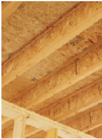
Engineered wood I-joists and OSB subflooring.
